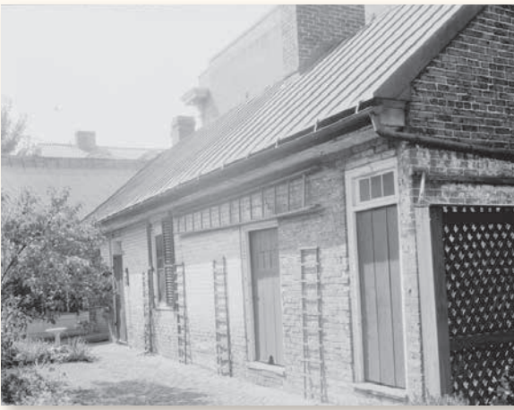
HABS photograph of the east elevation of the back building.
