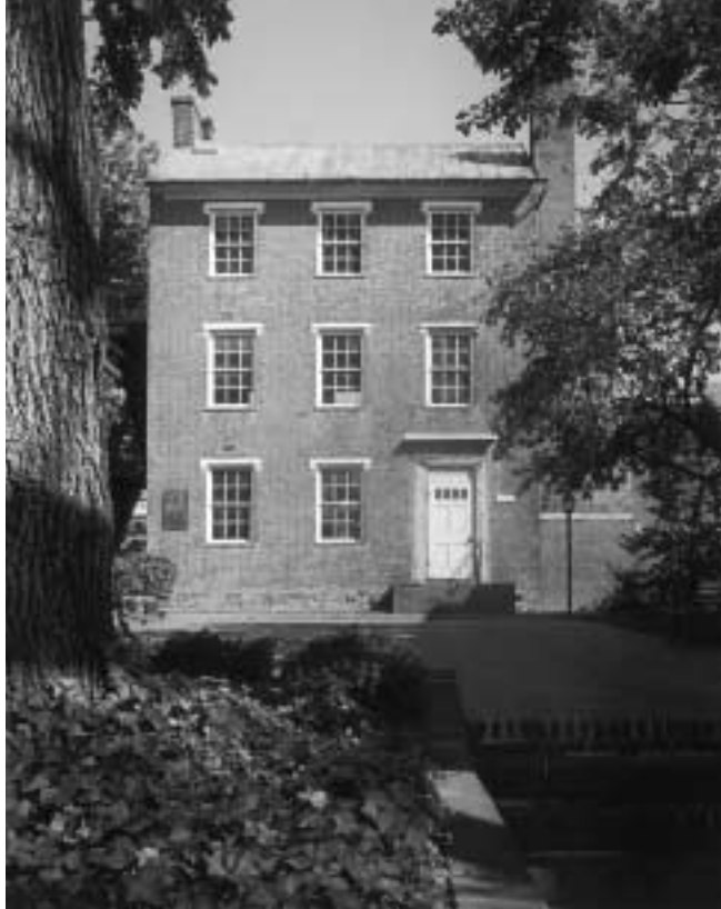
In the decades after its construction in 1785, the Alexandria Academy had acquired additional ornamentation around the windows and doorway. The $1.2 million dollar restoration undertaken by HAF returned this important early building to its original appearance and interior configuration. The Board of Trustees meets in the first floor classroom each month.
