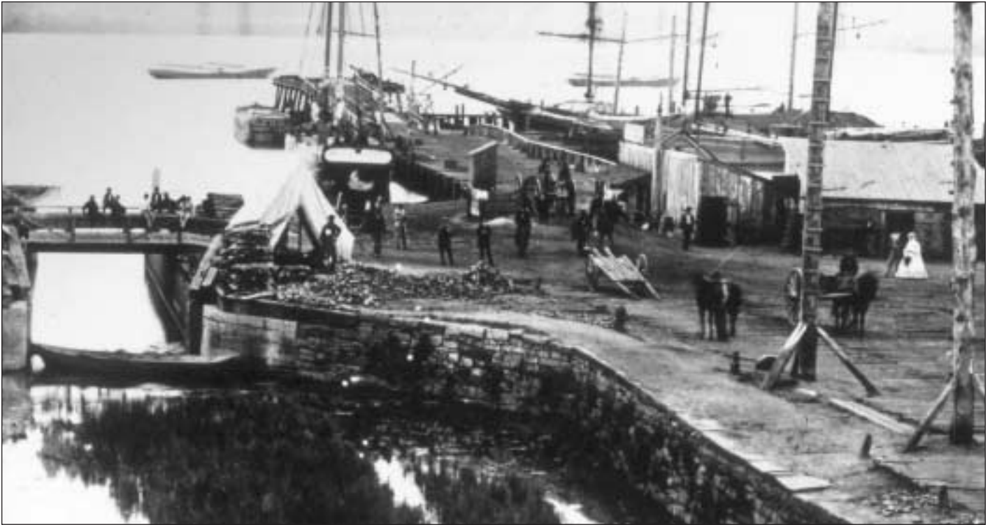
The tidal lock of the Alexandria Canal, which lowered barges into the Potomac, is captured in this early photograph. The canal, with its four locks and basins, was completed in 1845. This waterway connected the Chesapeake and Ohio Canal at Georgetown with the port of Alexandria via an aqueduct bridge. The tidal lock was excavated by Alexandria Archaeology in 1979.
