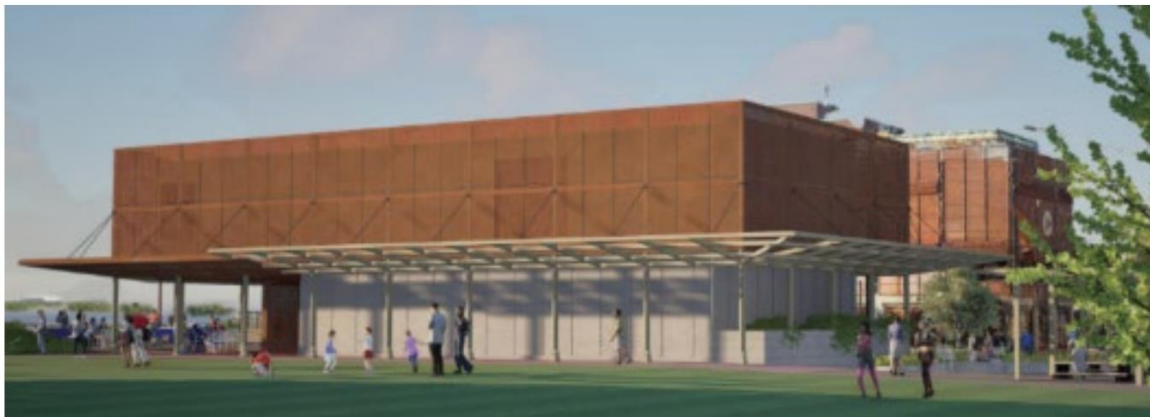
Figure 9: View of north side of Pump Station
